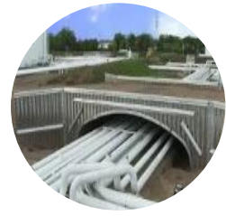
Inside Culvert, underground structure
