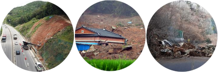
Roadside with steep slope, Landslide, Falling Rocks, Old Embankment & Bridge
